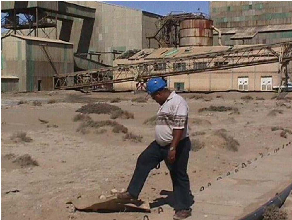
Roof in Background with Fragments Outside
