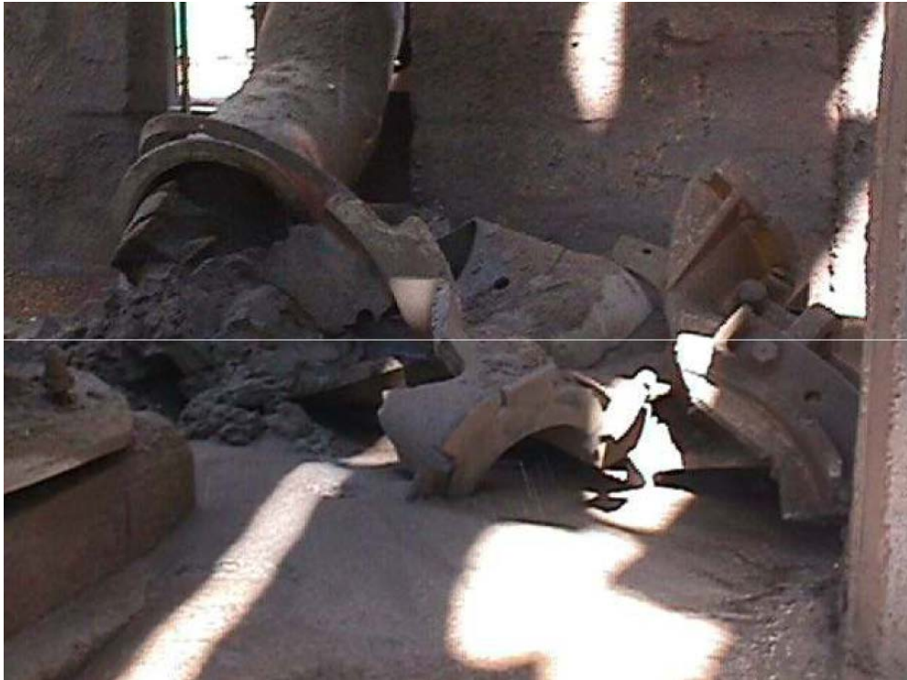
Remains of Pump in Pumphouse
